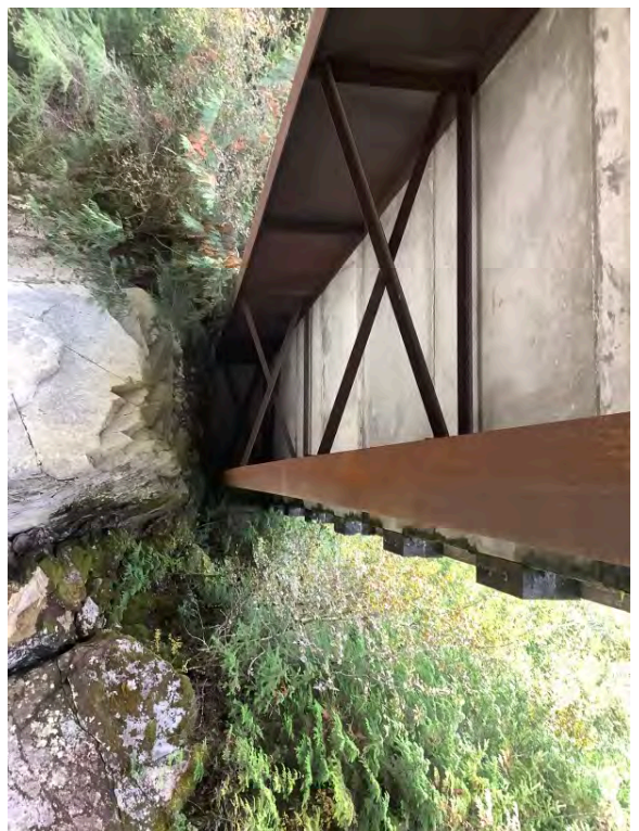
Right Bank Abutment when facing downstream
