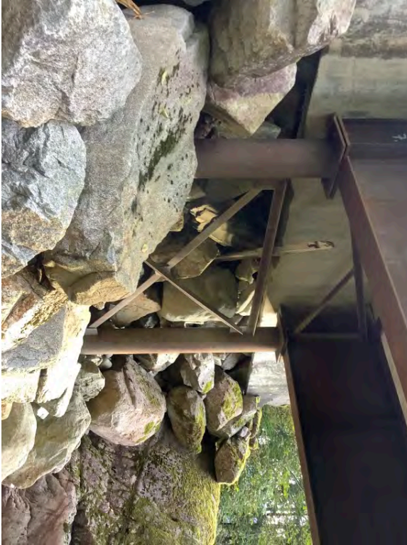
Left Bank Abutment when facing downstream
