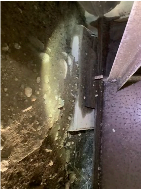
Right Bank Abutment when facing downstream - us side
