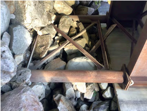
Left Bank Abutment when facing downstream
