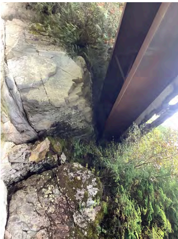
Right Bank Abutment when facing downstream
