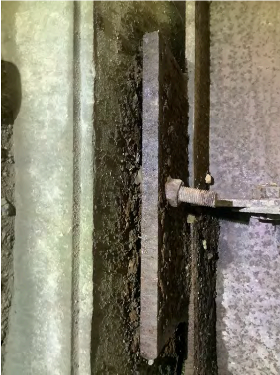
Right Bank Abutment when facing downstream - ds side
