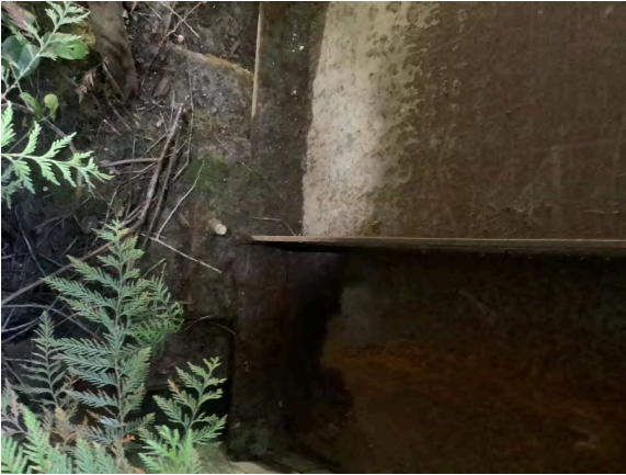
Right Bank Abutment when facing downstream
